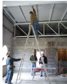
Installing the Ceiling Lamps
