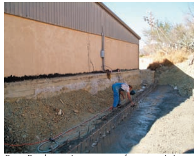
Pete Beal pouring cement for a retaining wall behind the library.
