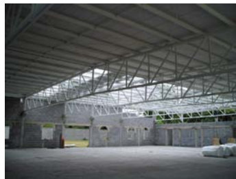
Interior of the multipurpose building
