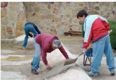
Volunteer Pete Beal and some students building a barrier.
