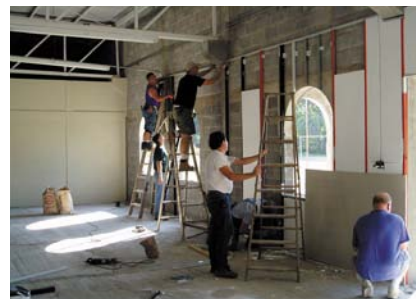
Work Group from Southwest Christian Church, Austin, Texas. Men installing the insulation in the Mexico Campus Multipurpose Building.
